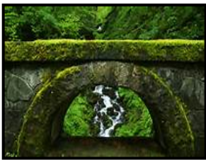
Moss on Bridge
